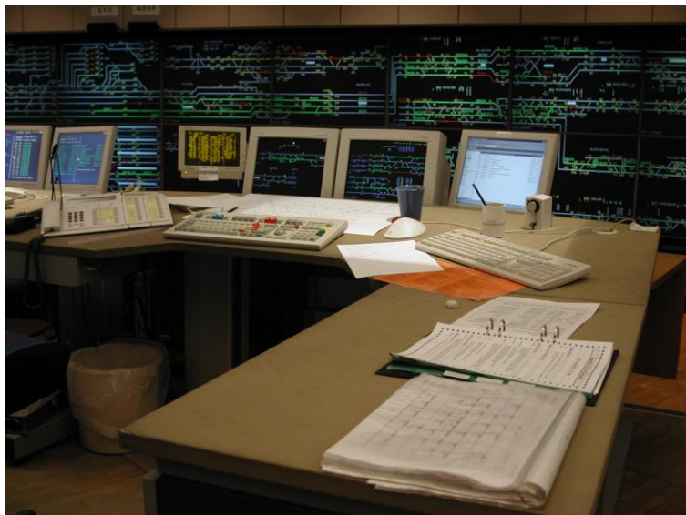
Fig. 1. Time-distance graphs on paper are a main tool in today's control of train traffic. The large panels on the walls are for tracking the trains' movement. Five other different systems shows required information for decision making about the traffic situation.
